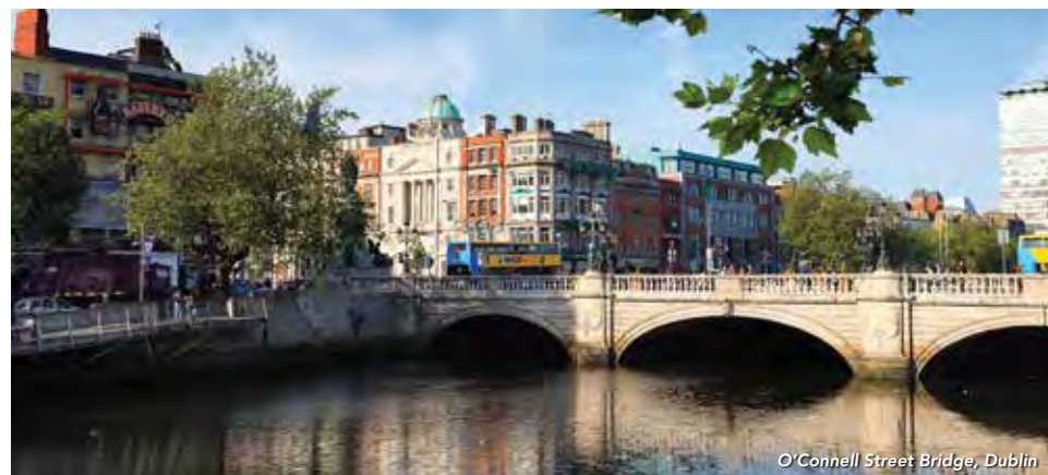
O'Connell Street Bridge, Dublin
